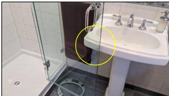
Glass door / Sink interference
